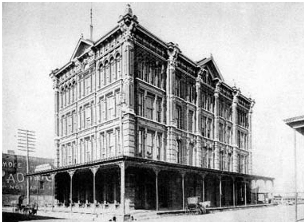
Moody Building, Galveston, Texas
